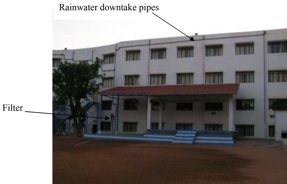
Underground pipes take the filtered rainwater to a dug well that is at the far end of the playground
