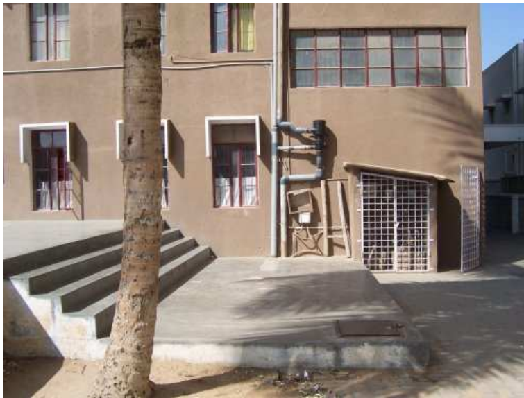
Water storage sump
